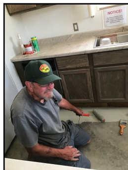
Bob Holman painting the WAPA kitchen floor with epoxy floor coating. Thank you, Bob.
