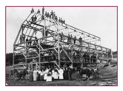
Ropes held by men kept the frame from tipping too far. After the parts were all tied together with the oak pins or the long bolts, the rafters were hoisted up and placed into position.
