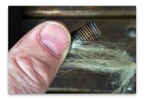
Hold the flax with y o u r t h u m b, bring it to the end of the pipe, and start wrapping in the direction of the threads.
