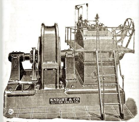
The accompanying cut shows the general arrangement of the KNIGHT WATER WHEEL, direct coupled to a 750 kilowatt generator, with governor mounted on top of wheel casing.
