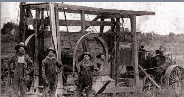
Robinson powered drilling rig
